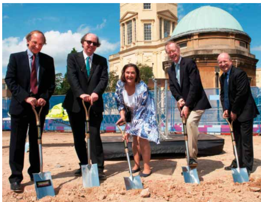
Work begins – pictured are Nick Woodhouse (former Head of Department), Sam Howison (Head of Department), Lavinia Clay (benefactor), Andrew Wiles, and Ewan McKendrick (University Registrar). 5
