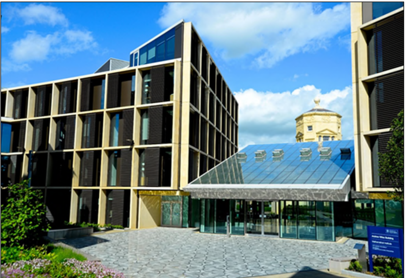
Figure 1: The Andrew Wiles Building
